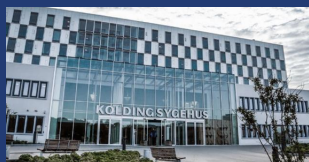
Kolding Hospital, Denmark Observational data following installation
