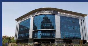
Air Forces Hospital, Egypt Observational data following installation
